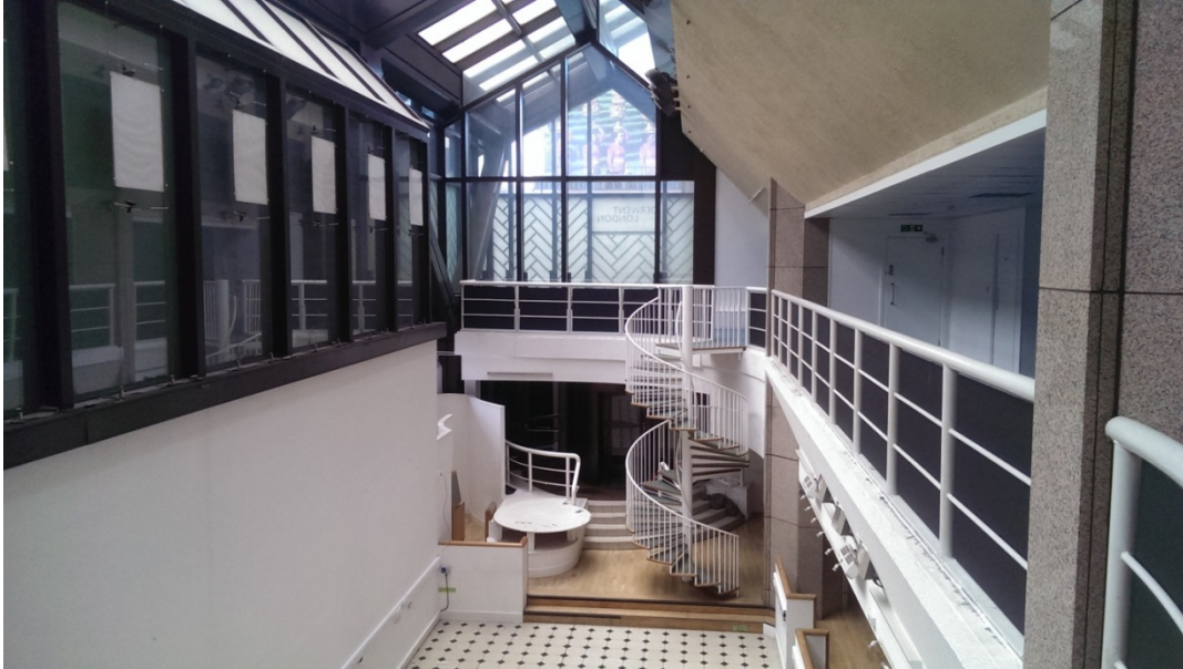
Figure 5 (a): Internal view of lean-to element taken from ground floor level
